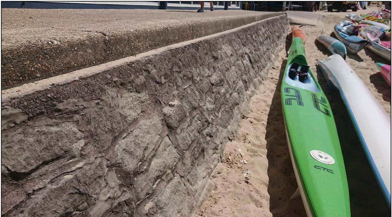
Figure 2.4 Photograph of existing seawall infrastructure
