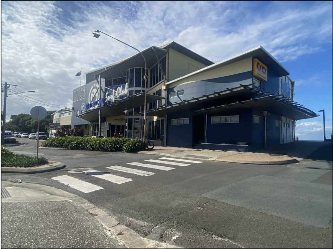
Figure 6 South-western corner of existing building looking north-east (Source: ASTP site visit 23 May 2024)
