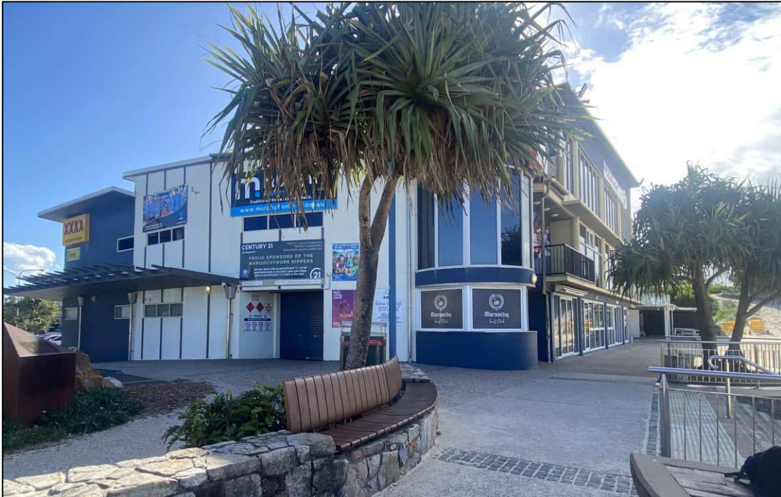
Figure 7 Southern edge of existing building looking north (Source: ASTP site visit 23 May 2024)
