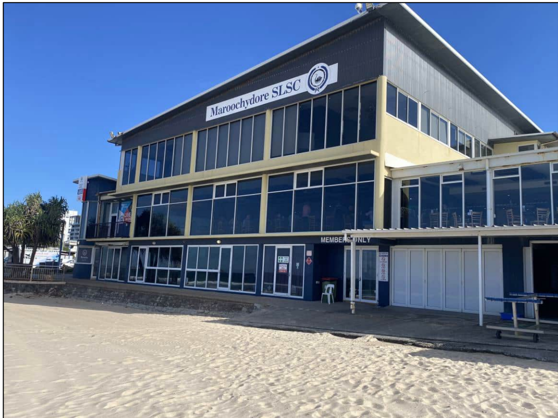
Figure 8 Eastern edge of existing building looking west (Source: ASTP site visit 23 May 2024)
