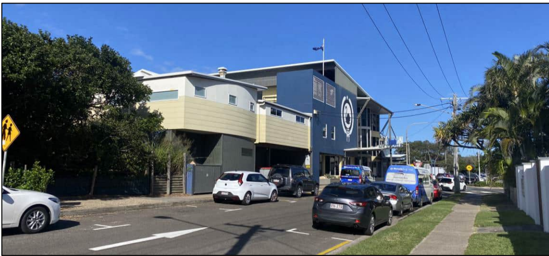
Figure 5 Western edge of existing building looking south-east (Source: ASTP site visit 23 May 2024)
